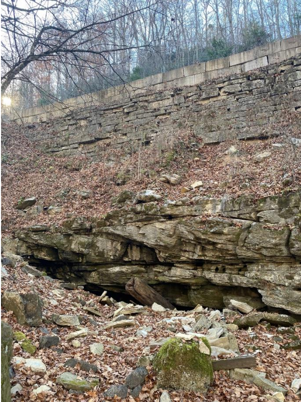
The creek entrance to Sinks – note the railroad bed foundation at the top.
