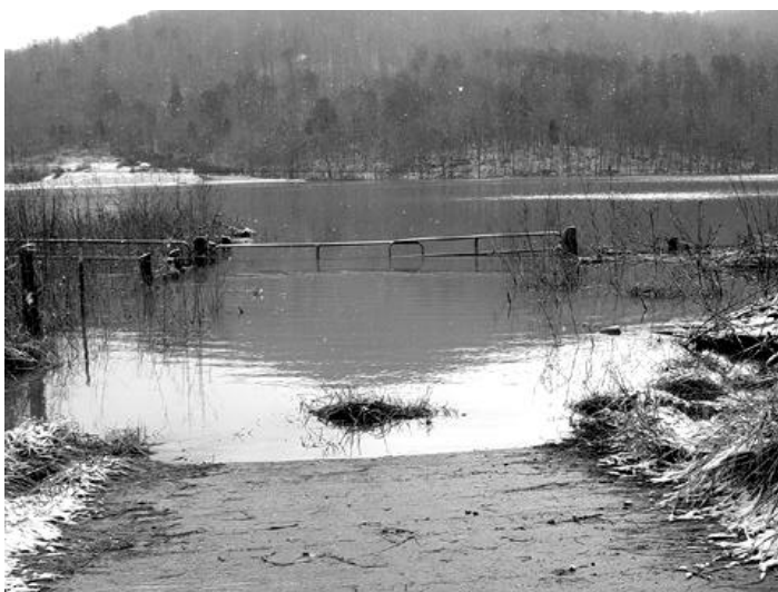
Note nearly submerged gate
